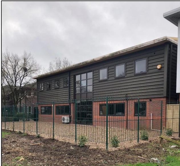
Front view from Reading Road
